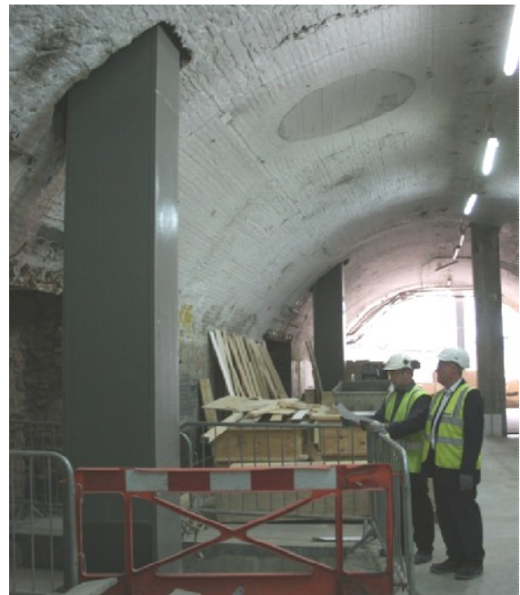
Figure 18 – New Columns on Micropile Bases
