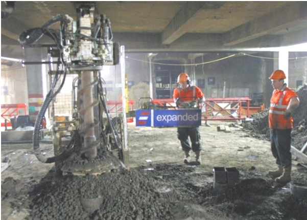
Figure 13 – Micropile boring using nominal 300mm diameter augers
