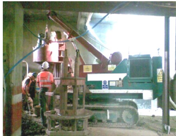
Figure 15 – Low headroom piling rig & crane
