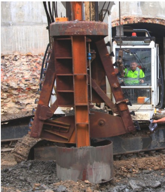
Figure 17 – Underream Tool
