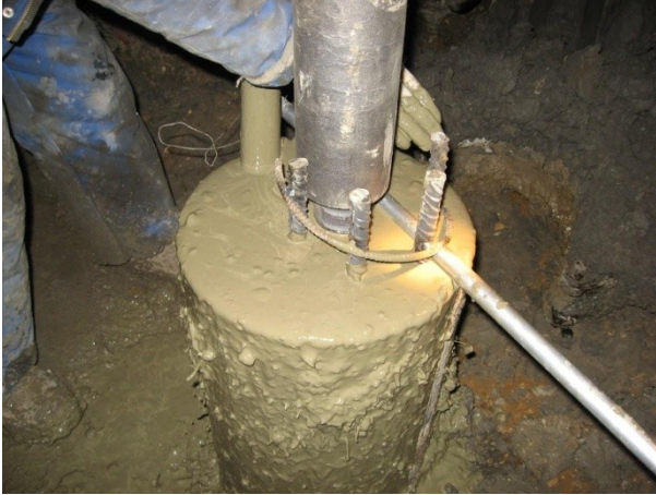
Figure 8 – Grouting of micropile (debris being flushed out)
