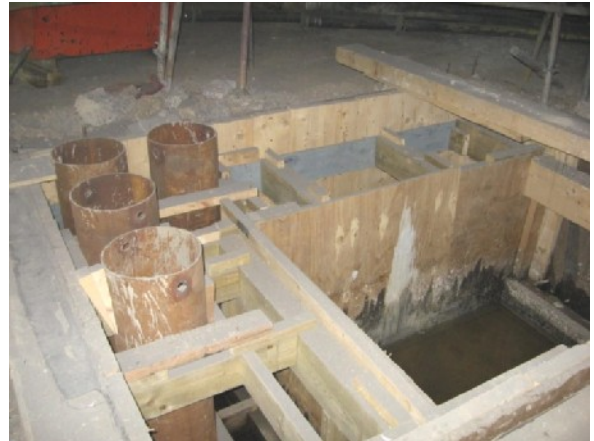
Figure 14 – Thin walled expendable steel casing
