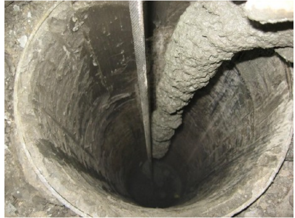
Figure 6 – Concreting of micropile
