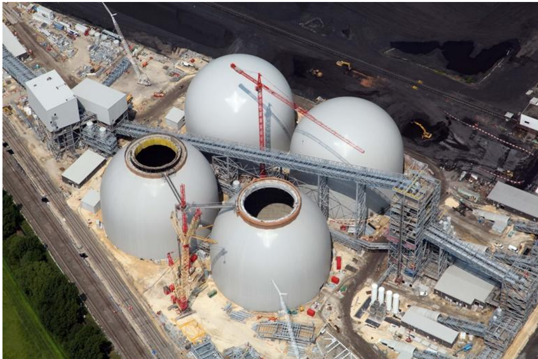
Four inflatable storage domes nearing completion
