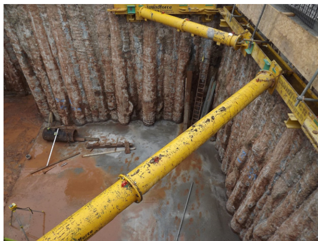
Figure 2. Out-of-position continuous flight auger bored secant piles
