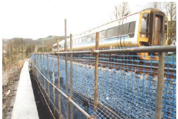
Figure (xviii) - Completed R/C Beam
