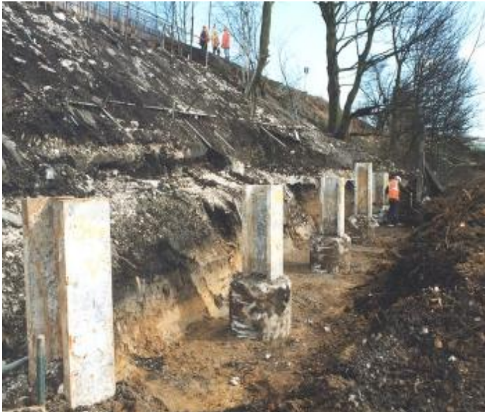
Figure(ix) - Trimmed Pin Piles
