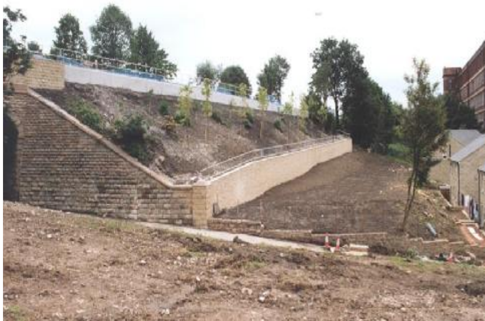
Figure (xx) - Completed Remedial Works
