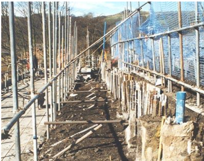
Figure (xv) - Tie Installation Complete
