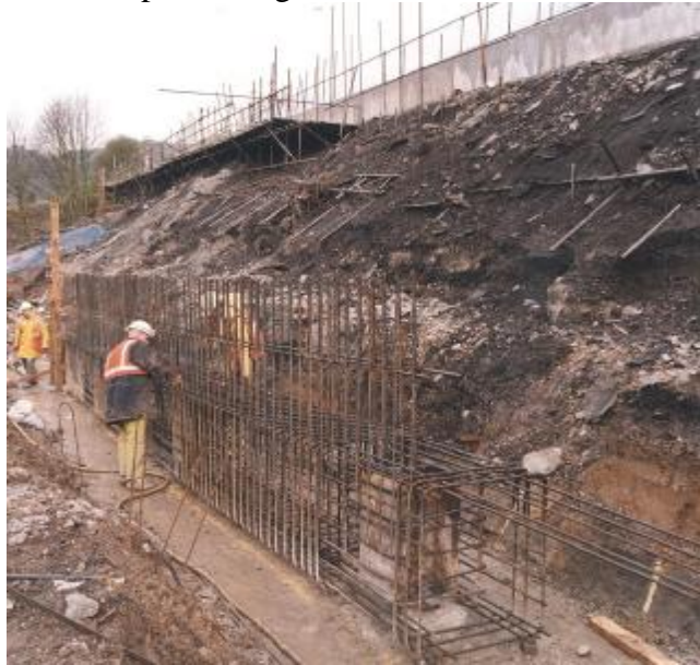
Figure(x) - Retaining Wall Reinforcement
