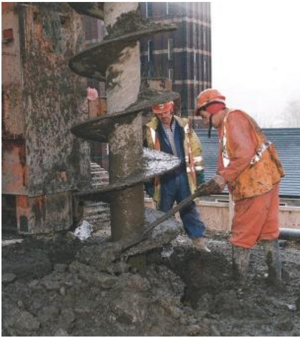
Figure (v) - Construction of 900 mm Diameter CFA piles
