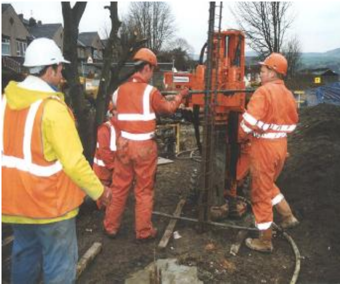
Figure (xii) - Installing Minipile Reinforcement
