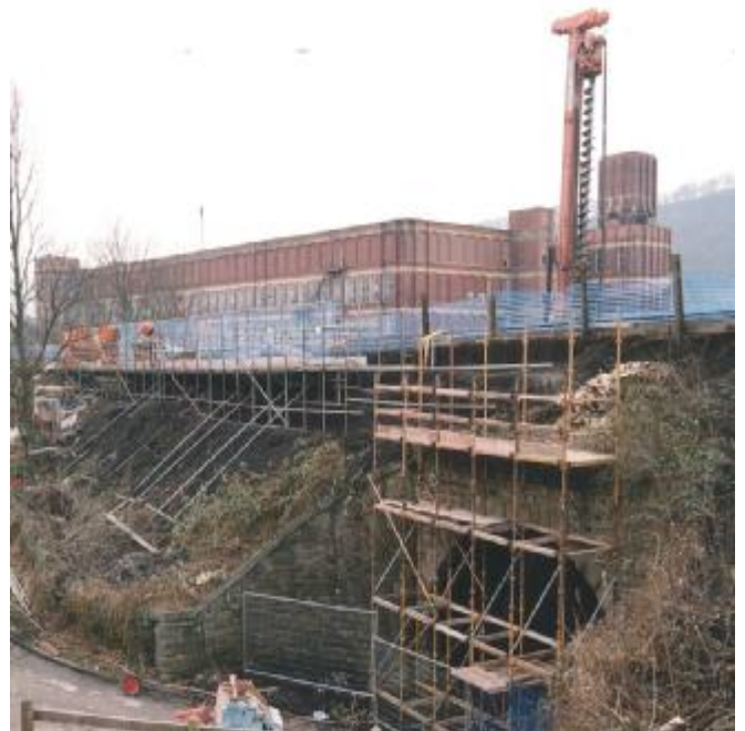
Figure (viii) - View looking South-East
