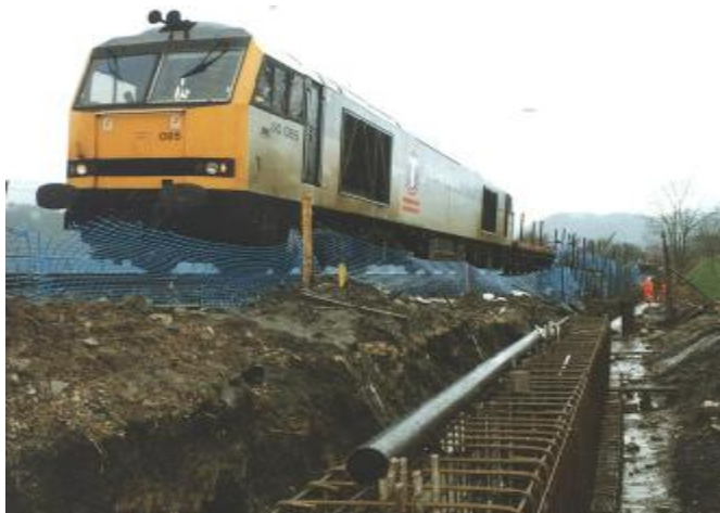
Figure (xvii) - Beam Reinforcement
