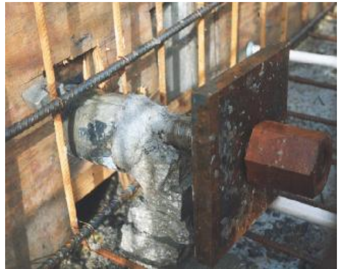
Figure (xvi) - Tie Bearing Plate
