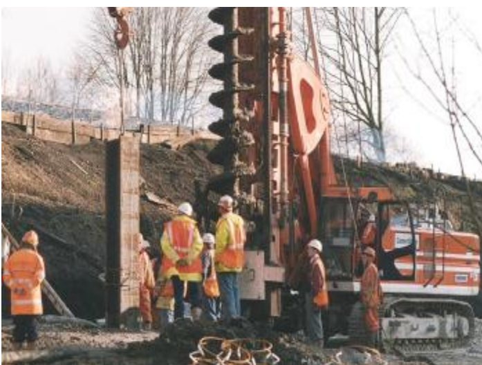
Figure (vii) - Installation of Universal Column
