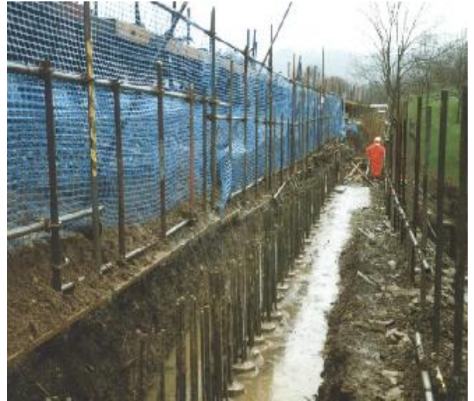
Figure (xiii) - Trimmed Minipiles
